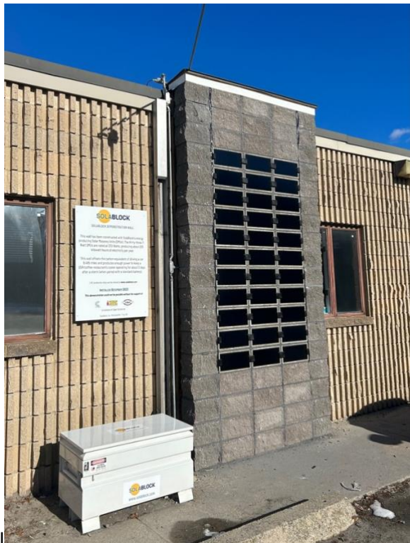
Image: SolaBlock’s SMU Test Wall in Chicopee MA
